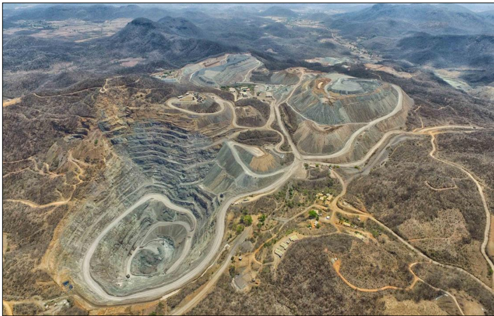
Figure 8 El Gallo Gold Site Photograph
