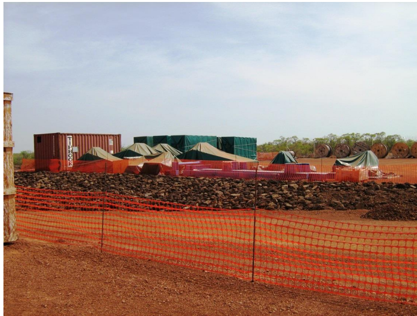
Figure 18-1: Typical Container Storage Area for Equipment and Materials
