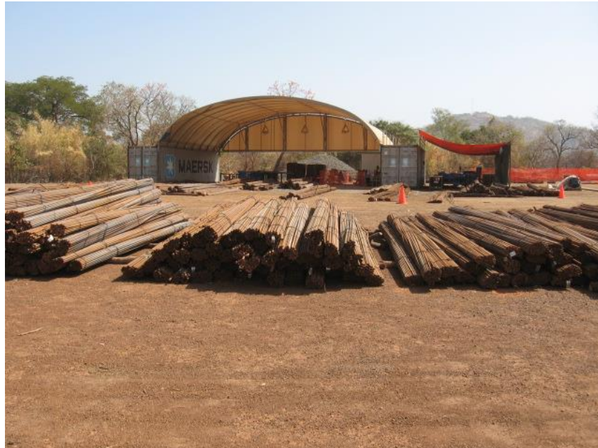
Figure 18-2: Typical Area for Storing Steel and for Rebar Bending
