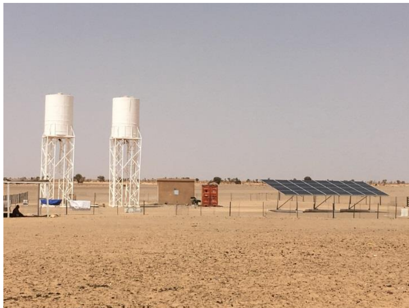
Figure 18-5: Typical Infrastructure for Deep Well Boreholes in the Region
