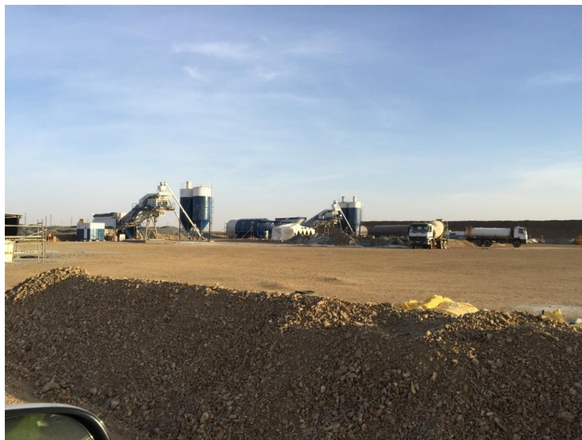
Figure 18-3: Typical Concrete Production Plant
