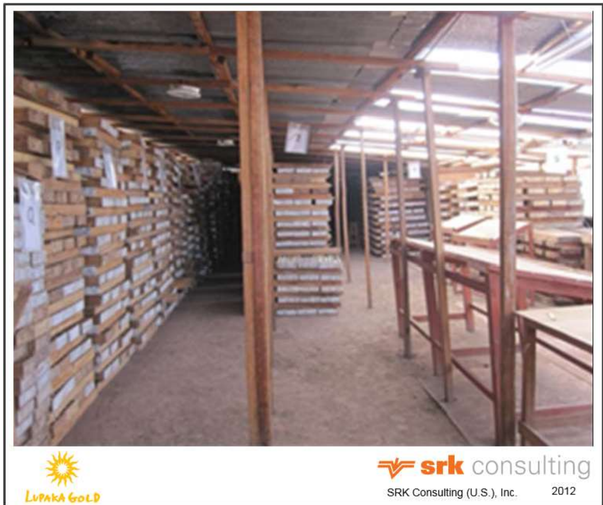
Figure 15: Invicta Gold Project Core Storage Building
