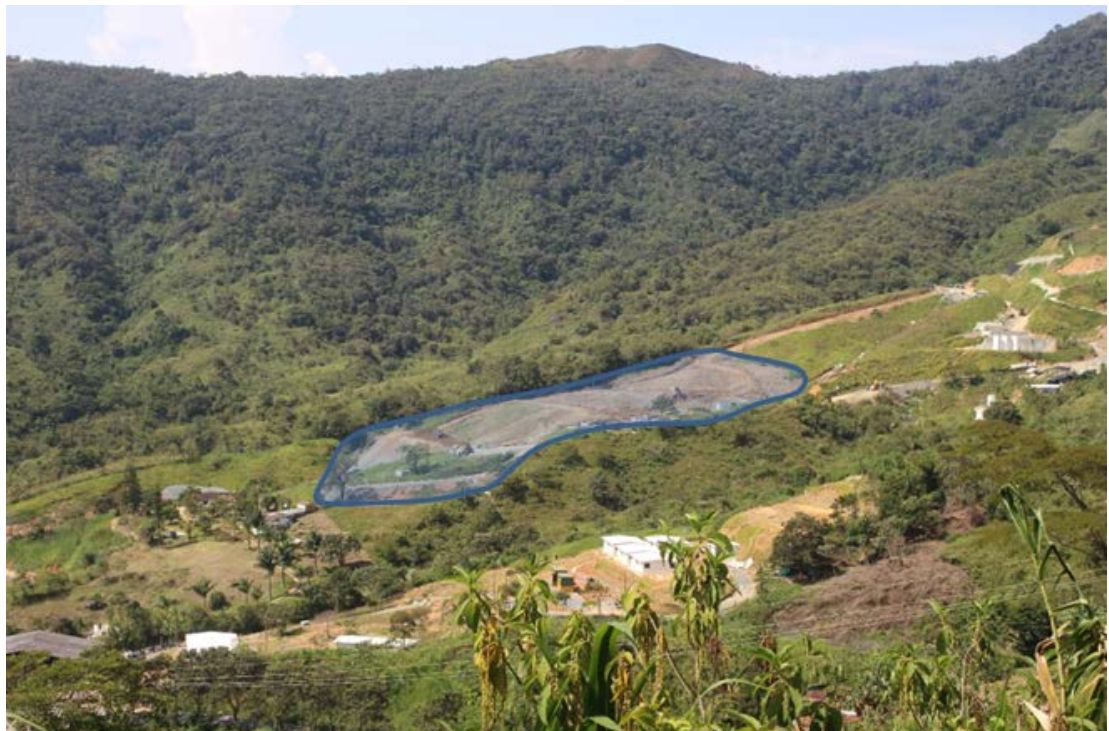
Photo 10: Waste Storage Facilities at Guayabito Area
