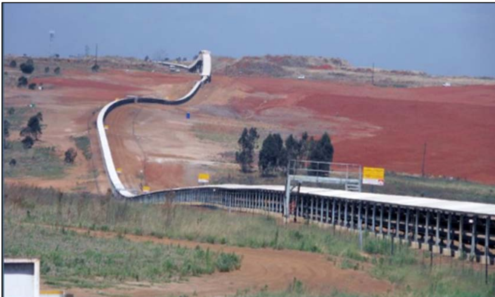
Figure 18-5: Curved Overland Conveyor (source: courtesy of ELB 2017)
