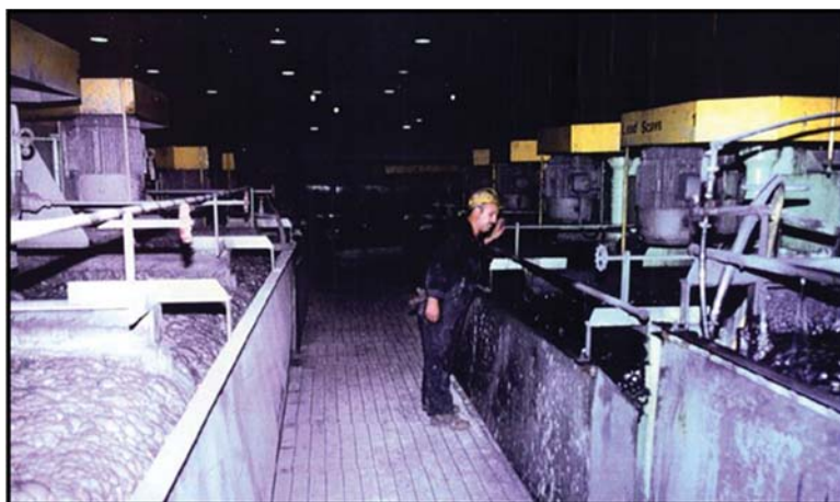
Figure 6-2: Flotation Circuit (circa 1990)
