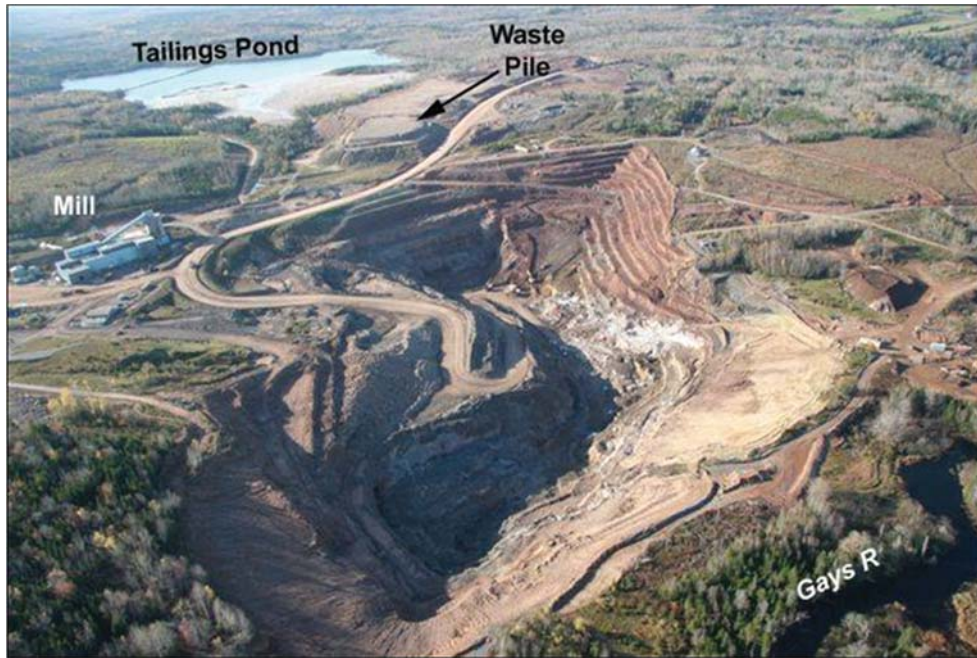
Figure 5-1: Site Infrastructure (Facing Southwest)
