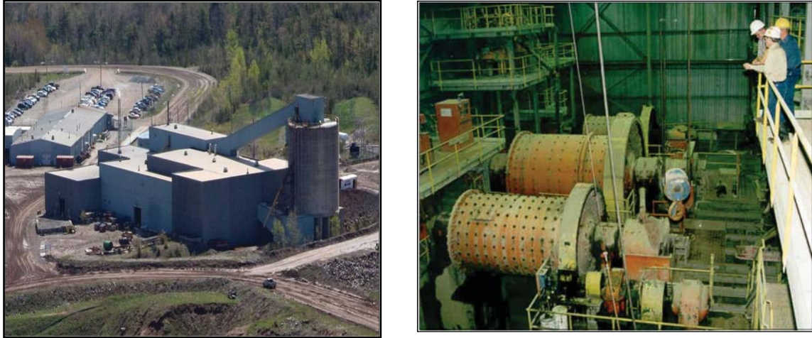
Figure 17-7: Views of the Outside and Inside (Right) of the Mill
