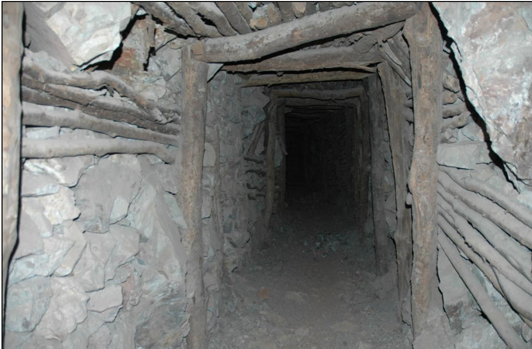
Photo 3 La Raya Vein System in the Bella Vista Tunnel: Timbering Extends for 10 metres across the Vein System (McBride Photo)
