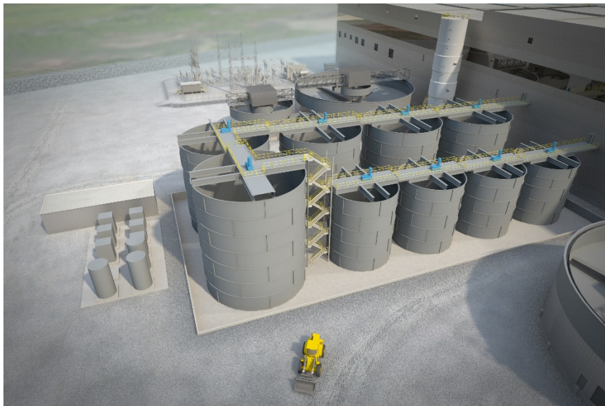
Figure 17-11: Configuration of the leach tanks
