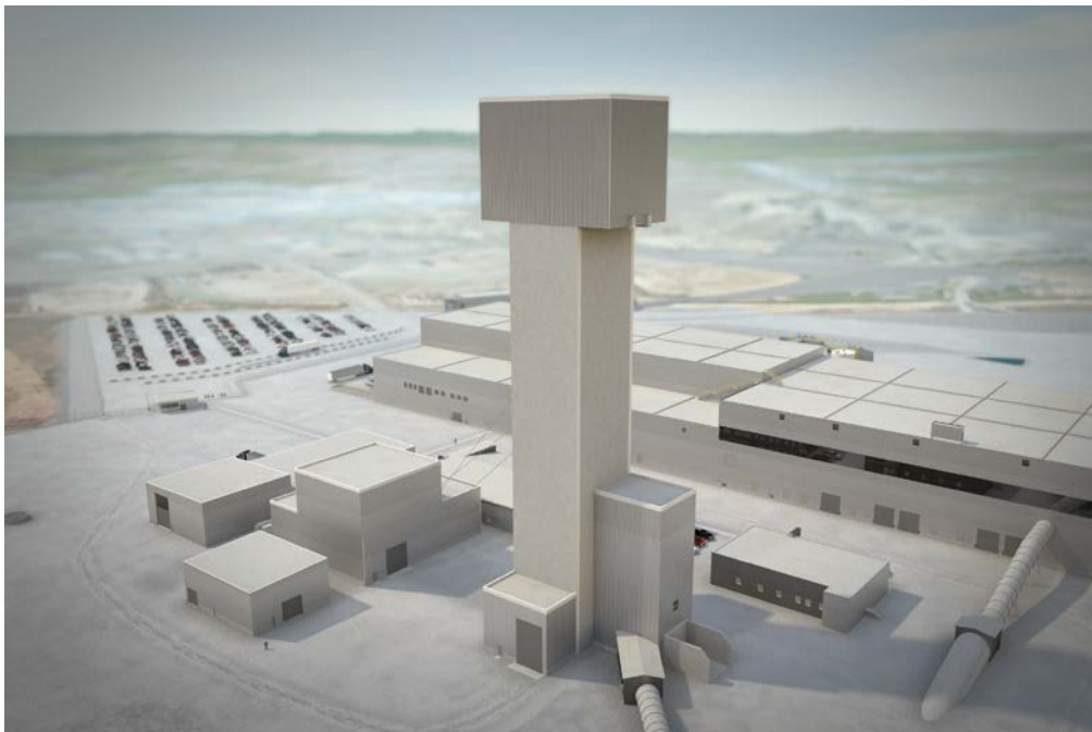
Figure 18-7: Headframe and hoist room buildings
