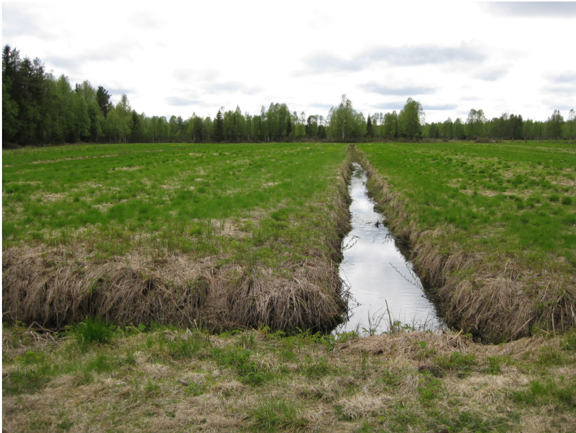
Figure 6. Drainage ditch in peat-covered areas at Foriet Property
