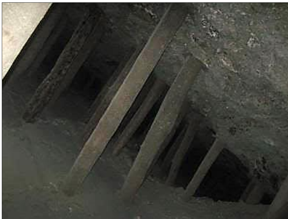
Figure 16-2 Open Stull Stope at Commodore Mine in Creede, Colorado
