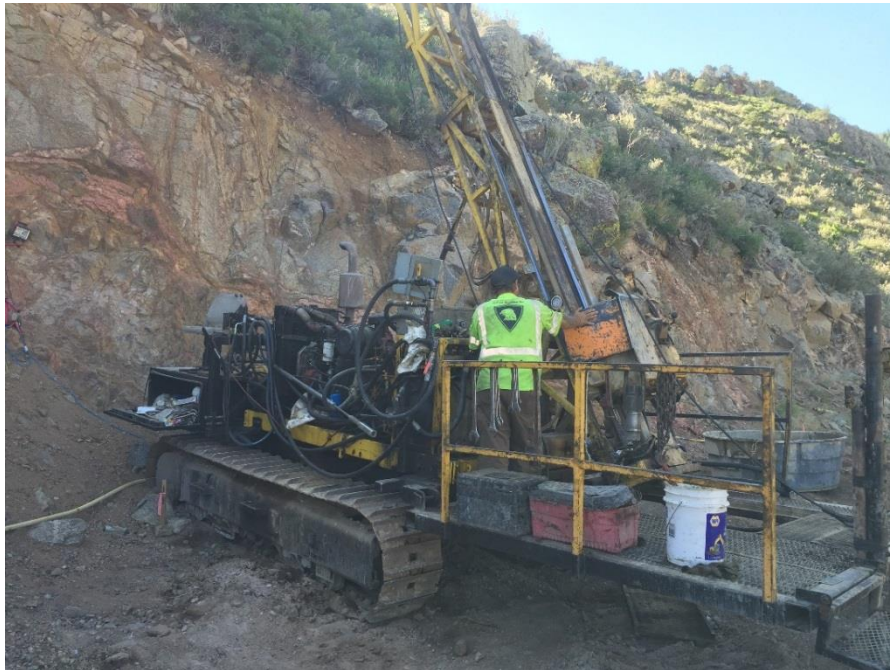
Figure 12.1: Godbe Drill Set-Up of Hole WG-16-34
