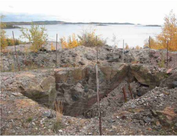
Fig. 9.14A Athona shaft. Although backfilled twice it continues to cave in, exposing the upper level of the shaft. The shaft is in amphibolite, although the dump (background) mainly has Athona granite.
