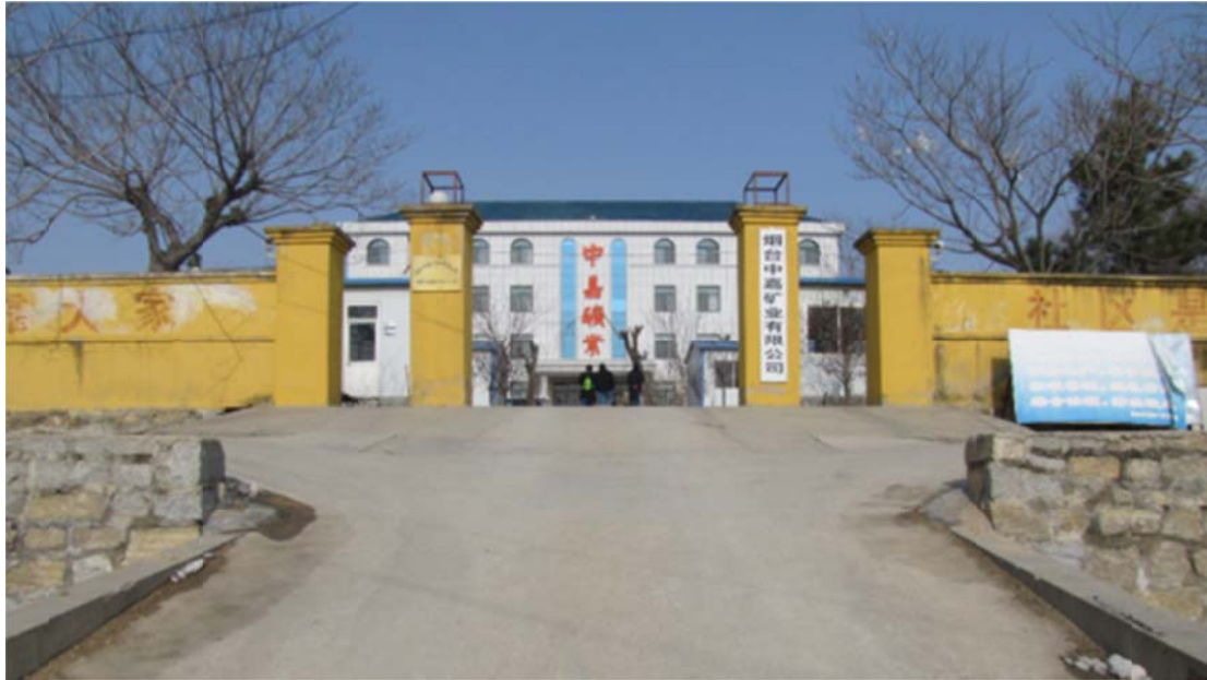
Figure 17-4: New Office Building
