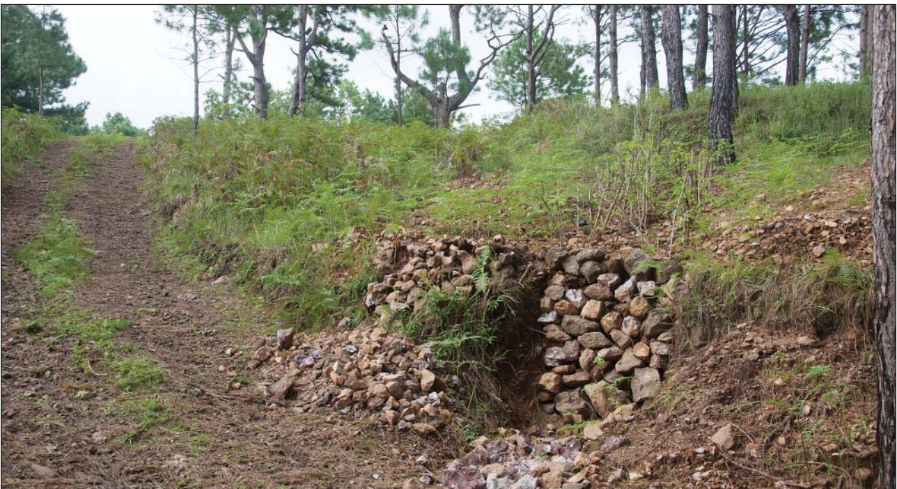
Figure 5: Rehabilitated ECR trench. Trenches were excavated using a small mechanical excavator and back-filled once sampling was complete. Back-filled trenches were re-vegetated.
